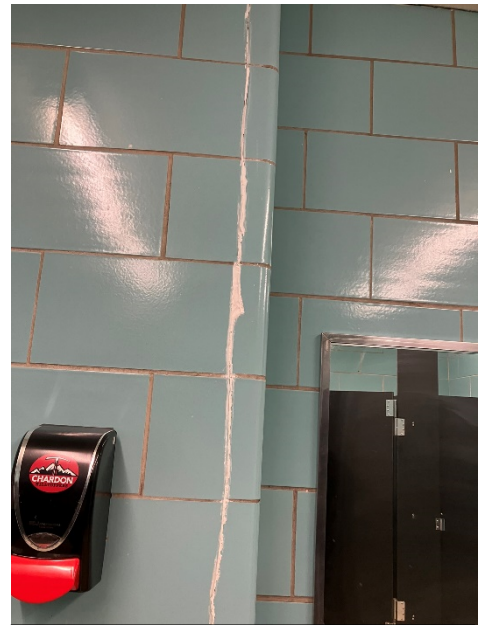
Interior wall cracks
