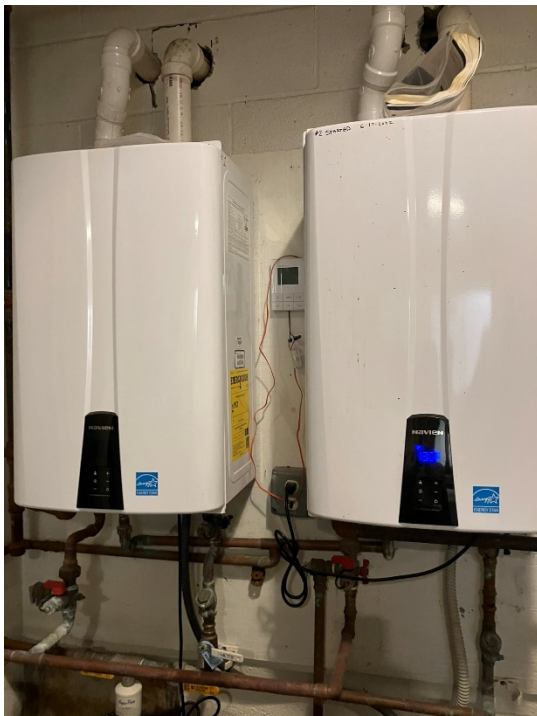
New kitchen tankless water heaters
