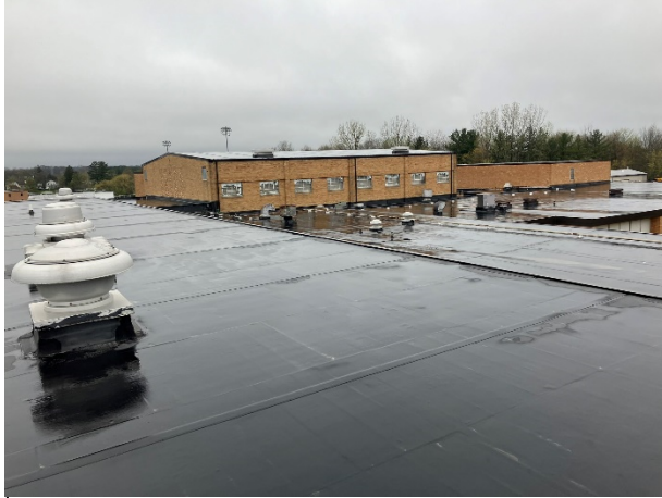
New EPDM roof system
