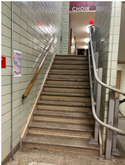
Stair handrail not compliant with current code
