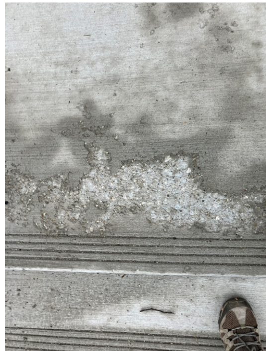
Spalling concrete
