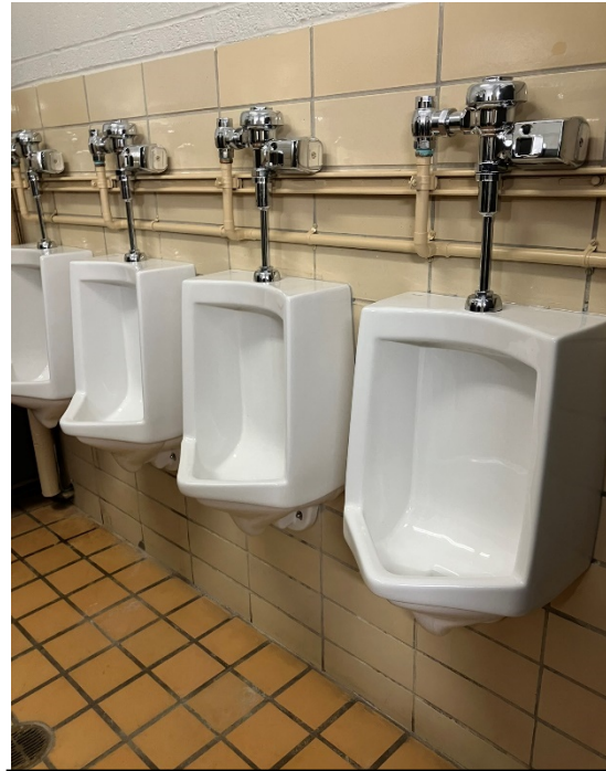
New auto flush valves on urinals
