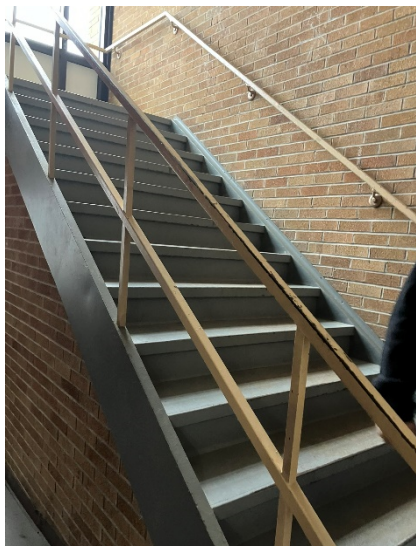
Stair handrail not compliant with current code
