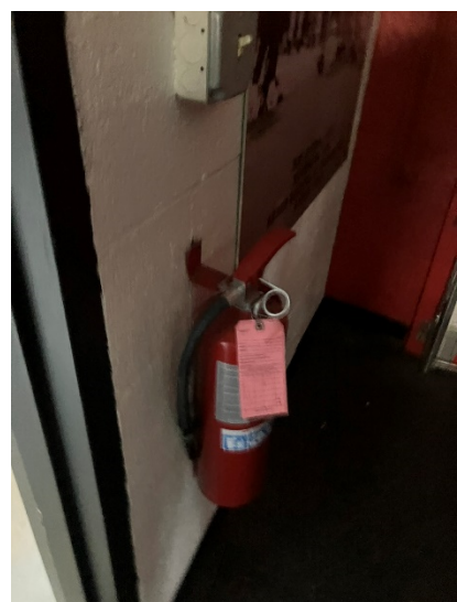
Fire extinguisher – not in wall cabinet
